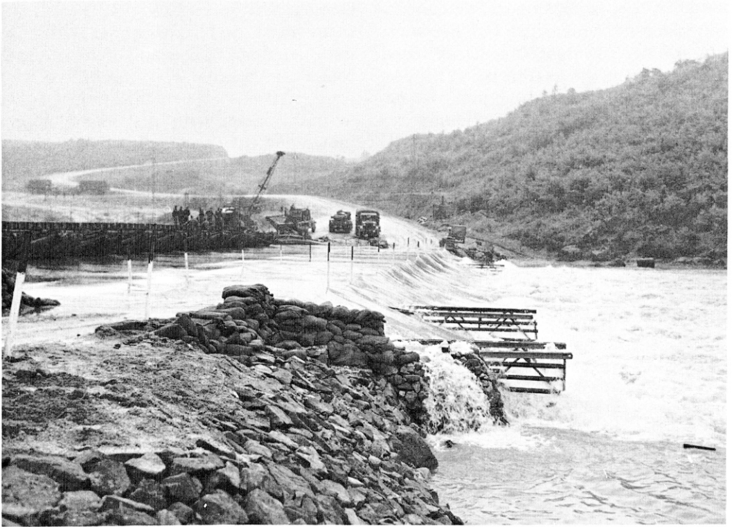
FLOODED BRIDGE CROSSING ON THE MAIN SUPPLY ROUTE, CH'ORWON VALLEY
